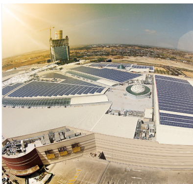
4.7 MW Johannesburg SSA Mall of Africa Commercial Solar Rooftop
